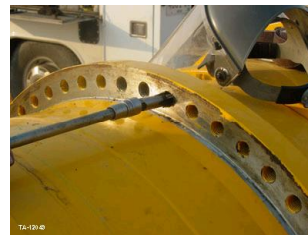
Cleaning paint and rust prior to torquing
